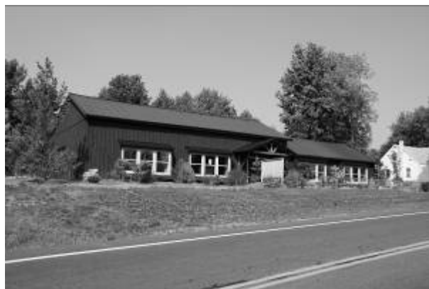
Former Walworth Town Barns on Penfield Road (photo 2007)
