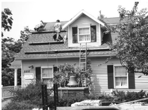
Museum roof being replaced
