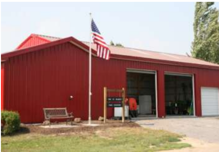
Walworth Town Park building 2.
