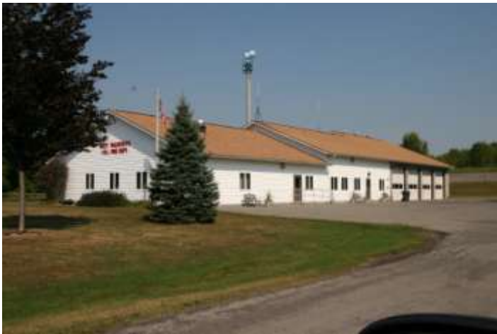
The West Walworth Fire Hall
