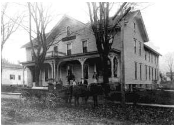
The Old Walworth Grange
