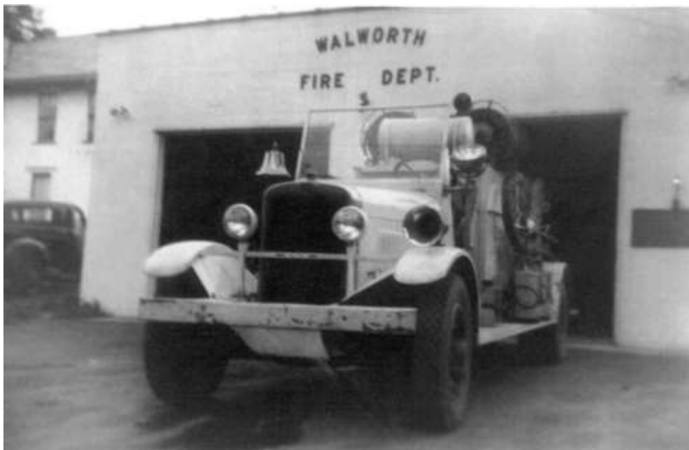
The second Walworth Fire Department building.
